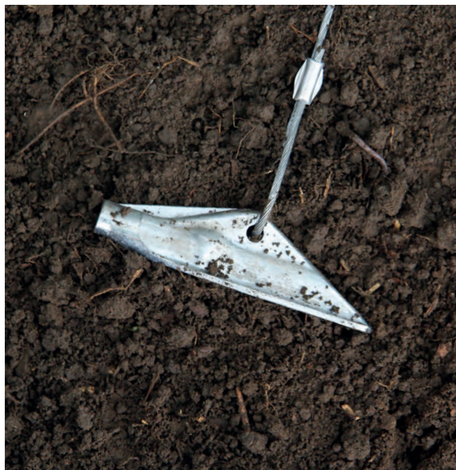
Anchor 3 - Activated and installed.
