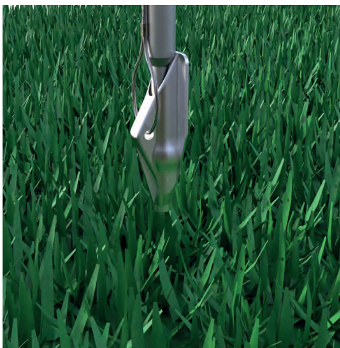
Anchor 3 being driven into the ground.
